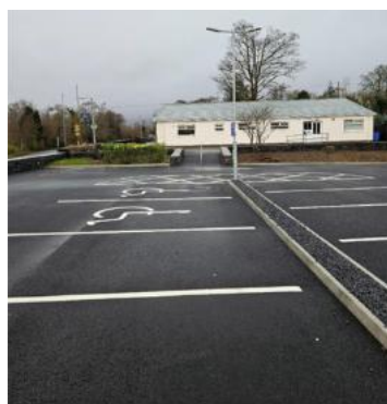
Public Car Park at Maam
