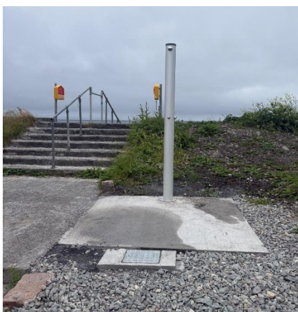
NEW OUTDOOR SHOWER INSTALLED BY DIRECT LABOUR STAFF AT TRÁ MHÓR, INDREABHÁN
