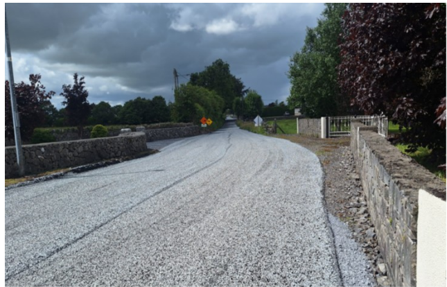
SURFACE DRESSING WORKS, CRUMLIN
