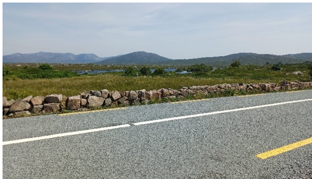
CS-RM-04 ROS MUC R340 ROAD – SURFACE DRESSED AND LINED
