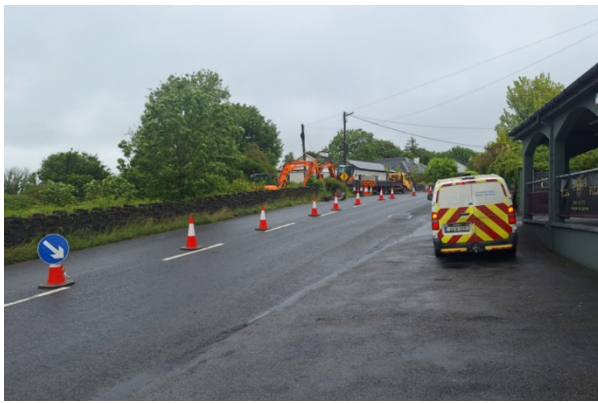
CORRUNDULLA DRAINAGE WORKS,
