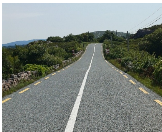
CS-RM-04 ROS MUC R340 ROAD – SURFACE DRESSED AND LINED
