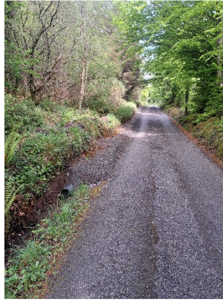
KILCRIMPLE VERGE REPAIR, LANNAGHT
