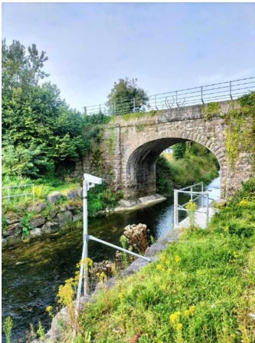
Figure 2-1: OPW Hydrometric Station Craughwell 29007 (facing downstream)
