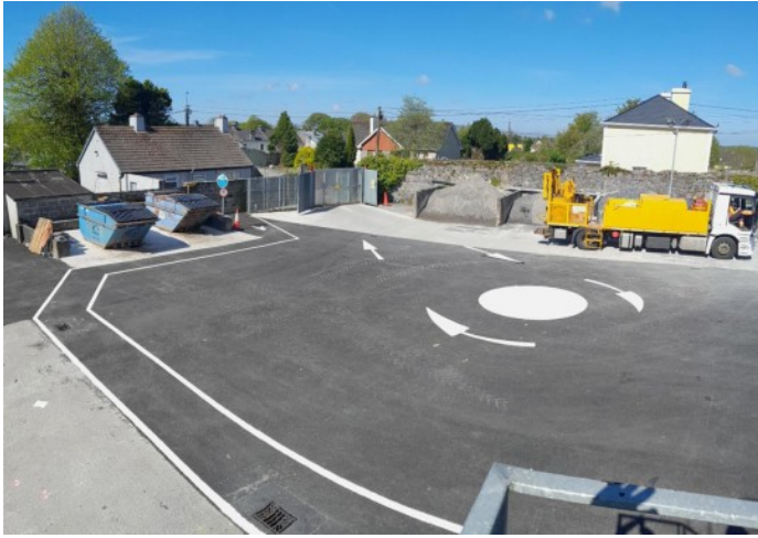
GORT ROADS DEPOT – INSTALLATION OF ROAD MARKINGS TO ENHANCE SAFETY
