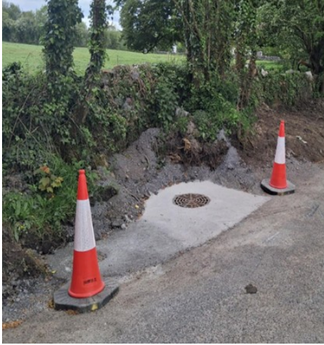
DRAINAGE WORKS @ MONEYTEIGUE
