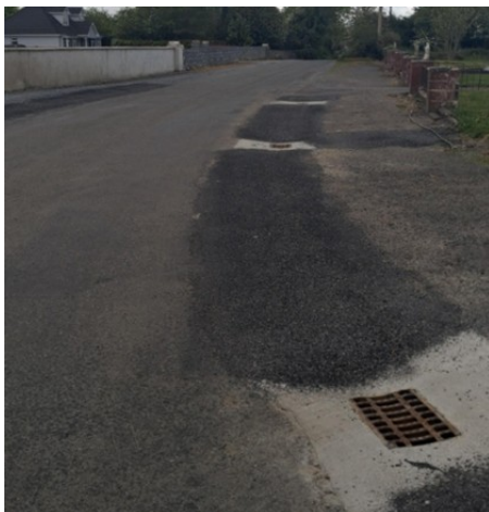
DRAINAGE WORKS @ CAHERNAFINISKER
