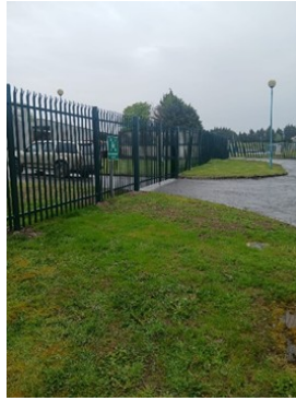
LOUGHREA ROADS DEPOT - NEWLY INSTALLED SECURITY FENCING AND CONCRETE APRON AT STORAGE/LOADING BAYS
