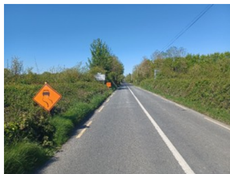
ROAD RESURFACING AT R352 CLONCO
