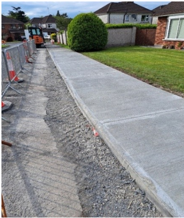
FOOTPATH REPAIR WORKS AT HAWTHORN ESTATE, BALLINASLOE
