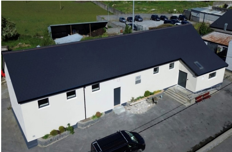
KILLERERIN COMMUNITY CENTRE, BARNADERG, COMPLETION OF RE-ROOFING, MAY 2026 FUNDED BY THE CLÁR PROGRAMME
