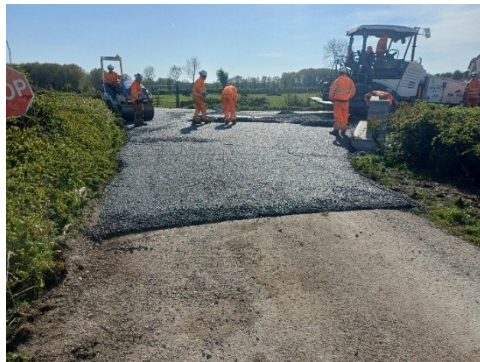
OVERLAY WORKS AT KILMURRY, KILLIMOR ON THE L4314
