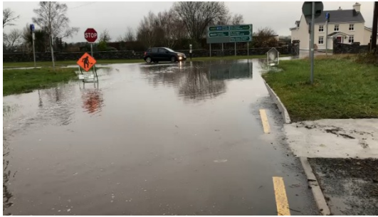
BEFORE WORKS COMMENCED
