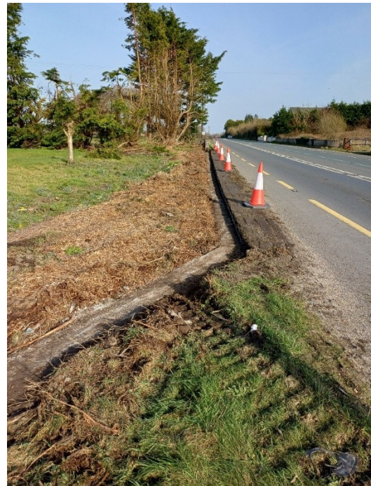
RECONSTRUCTION OF DAMAGED BOUNDARY WALL ALONG THE R446 AT CAHER CROSS
