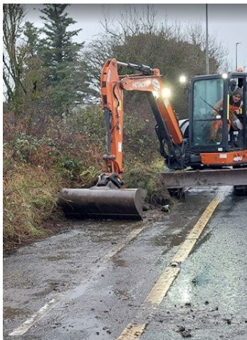
VERGE MAINTANENCE WORK – REGIONAL ROADS
