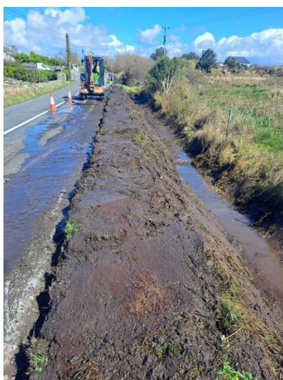
DRAINAGE WORKS BEING UNDERTAKEN BY DIRECT LABOUR STAFF ALONG THE AN SPIDÉAL TO MAIGH CUILINN ROAD
