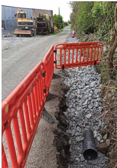
DRAINAGE WORKS @ CAHERFINISKER
