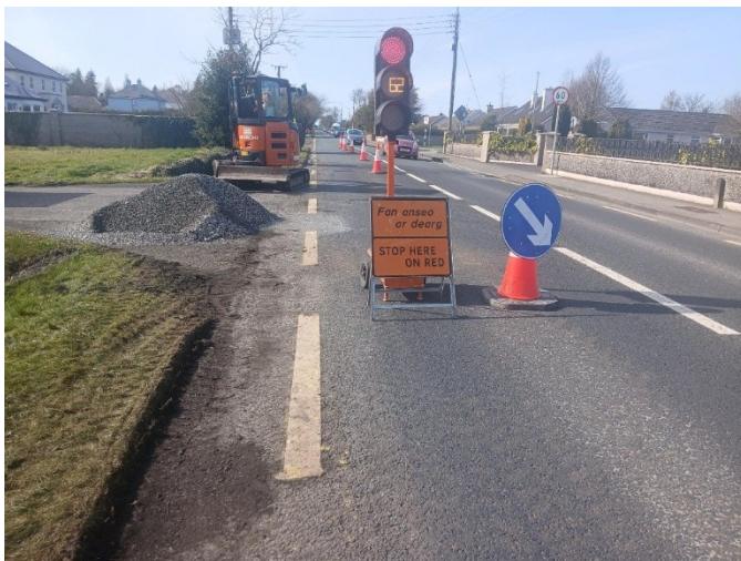
DRAIN CLEANING WORKS ON N63 MOUNTBELLEW
