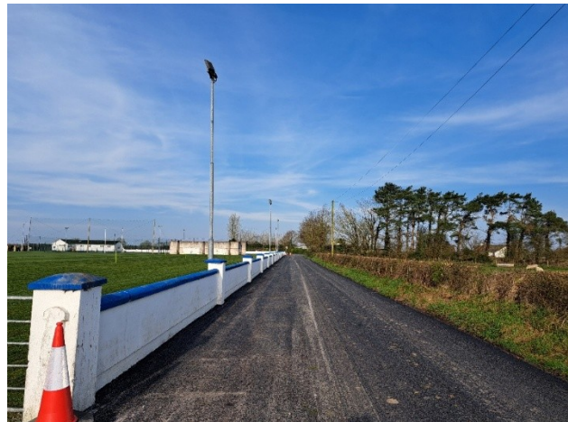
OVERLAY OF THE L-8726 AT BALLINAKILL, EYRECOURT UNDER RESTORATIVE IMPROVEMENT WORKS PROGRAMME 2026
