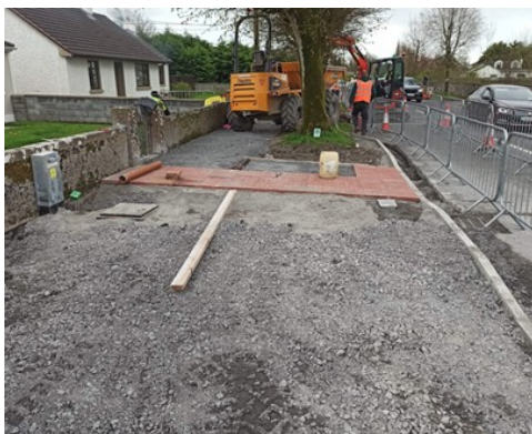
FOOTPATH REPAIRS, ORANMORE
