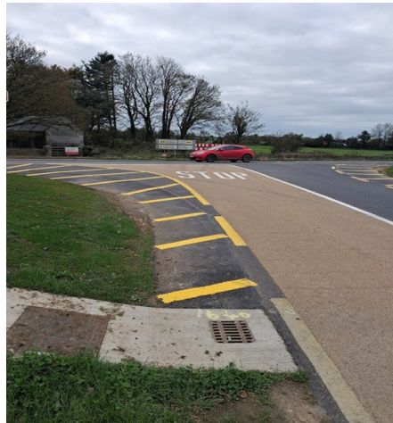
DERRYDONNELL CROSS IMPROVEMENT WORK
