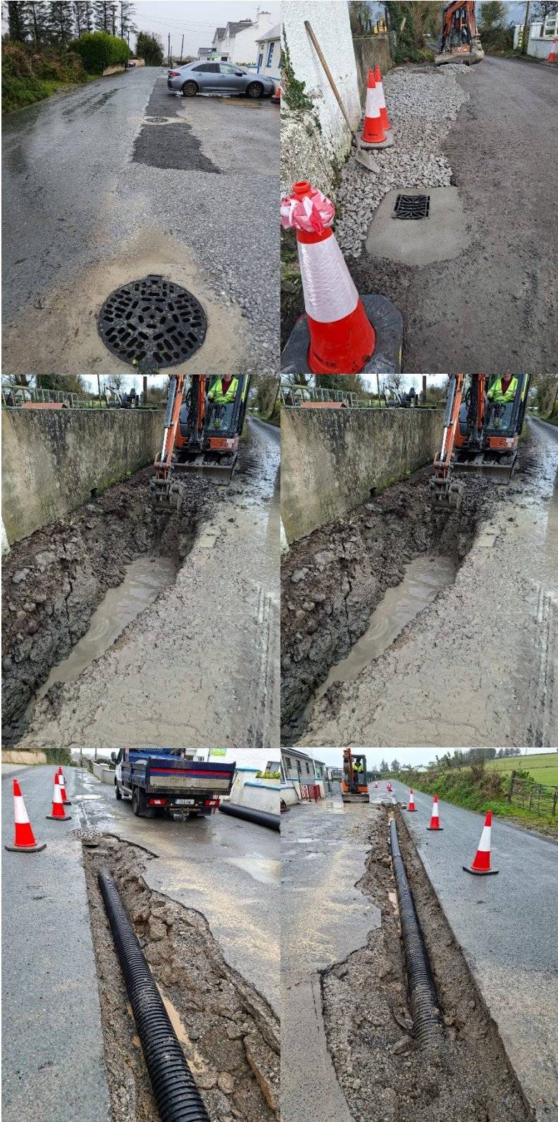
DRAINAGE WORKS – KILLEENADEEMA NATIONAL SCHOOL
