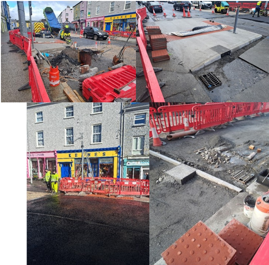
LOW-COST SAFETY IMPROVEMENT PROJECT ADDRESSING ROAD SAFETY CONCERNS AT THE PEDESTRIAN CROSSING, GORT
