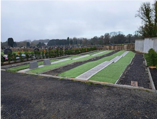
CONSTRUCTION WORKS FOR THE URN PLOTS AT CREAGH CEMETERY
