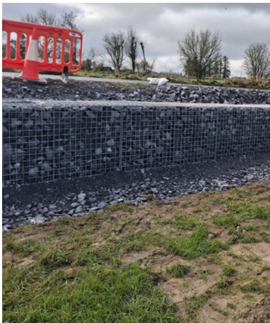
RETAINING WALL - COOLARNE
