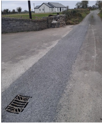
MCDONALDS LANE, ATHENRY – FOOTPATH REPLACEMENT DRAINAGE WORKS – GORTROE, COR AN DOLA
