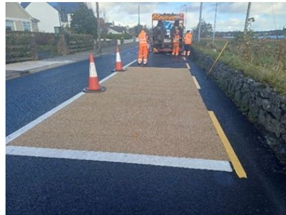
REINSTATEMENT OF HIGH FRICTION SURFACING AT PEDESTRIAN CROSSING ON R380
