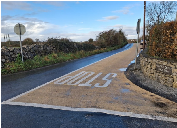
SAFETY IMPROVEMENT WORKS – CASEY'S CROSS
