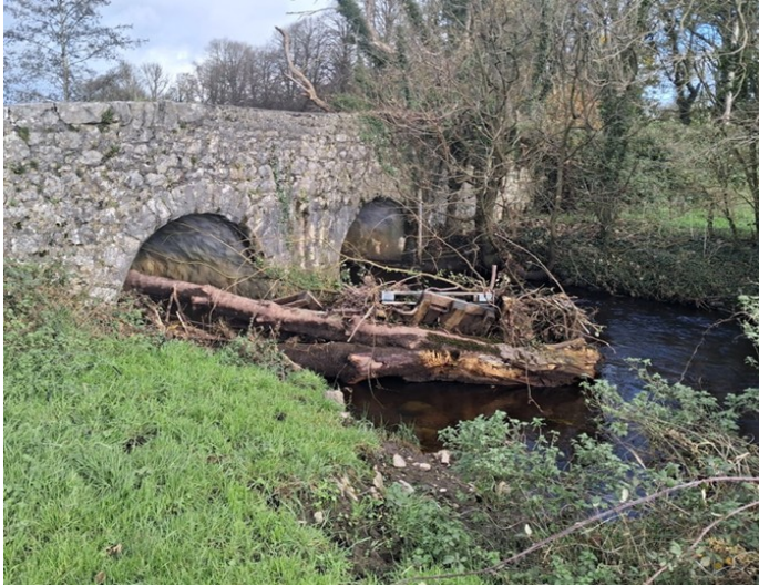
SAFETY IMPROVEMENT @ CARNMORE ONGONG MAINTENANCE OF CLARIN RIVER – MULPIT
