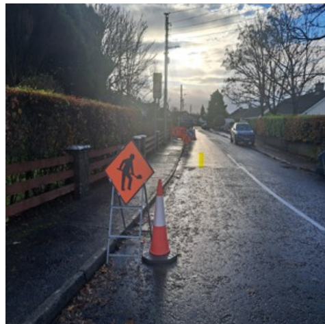
NOTICE OF MOTION FUNDED FOOTPATH IMPROVEMENT WORKS AT BEECHGROVE, ORANMORE
