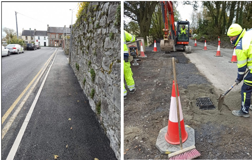
COURT LANE, ATHENRY – FOOTPATH REPLACEMENT DRAINAGE WORKS – RYEHILL
