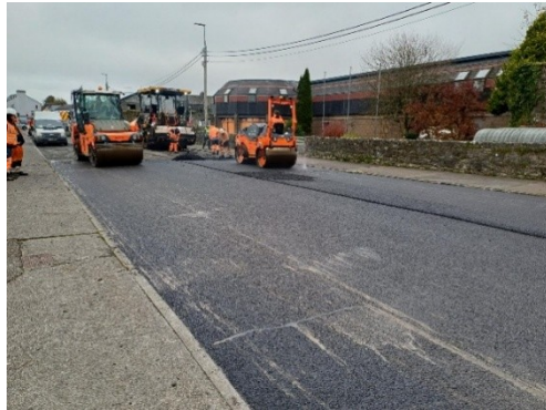
OVERLAY WORKS AT THE R380/R351 JUNCTION IN LOUGHREA TOWN
