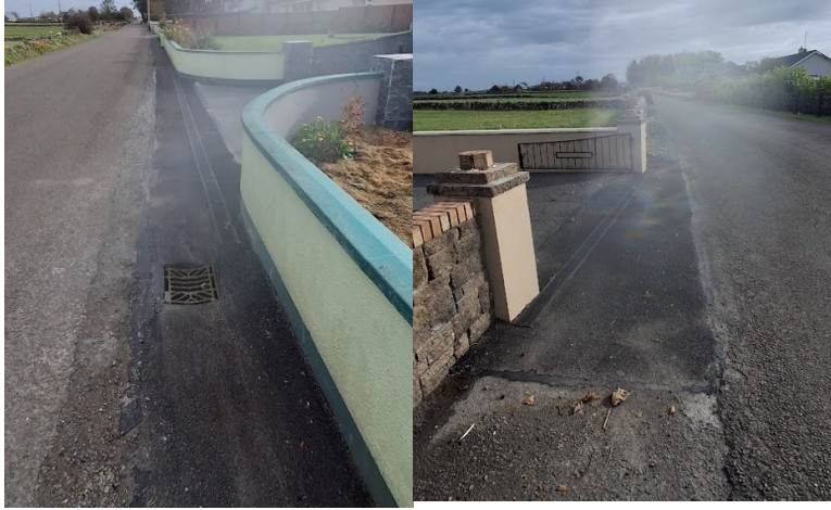
FLOOD RELIEF WORKS AT BALLINVOHER
