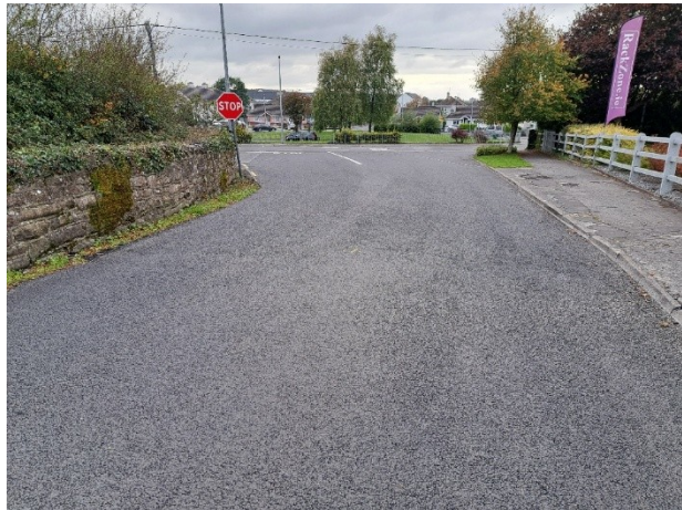
ROAD INLAY WORKS ON-GOING ON THE L-4603 AT POOLBOY, BALLINASLOE
