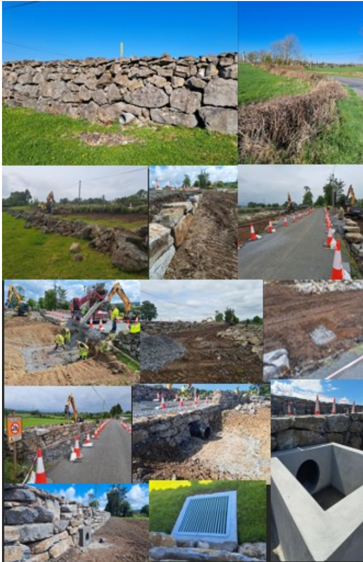
ROAD RAISING PROJECT AT GRANNAGH
