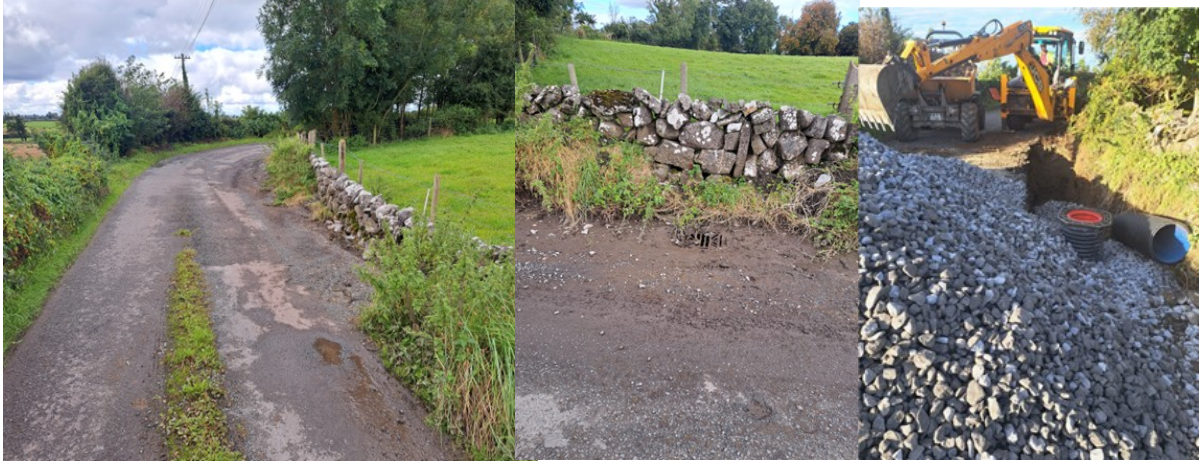
DRAINAGE AT RATHBAUN FARM
