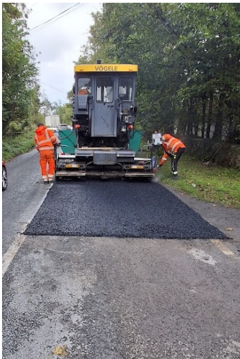
RESURFACING AT BAUNMORE
