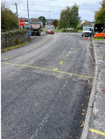
ROAD INLAY WORKS COMPLETED ON THE R348 SARFIELD ROAD, BALLINASLOE
