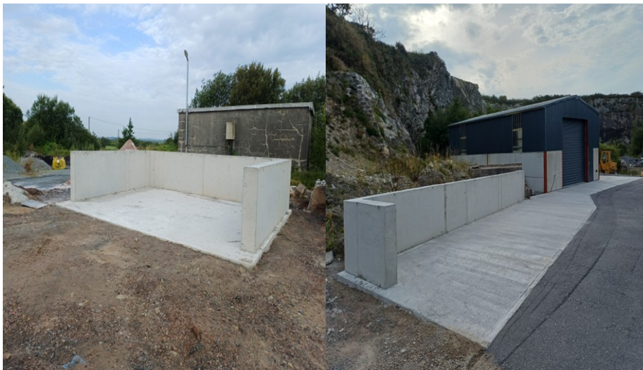
STATIC RISK ASSESSMENT WORKS RECENTLY UNDERTAKEN IN TONABROCKY
