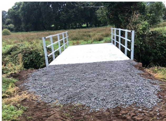
LAND ACCOMMODATION BRIDGE AT KILCHREEST
