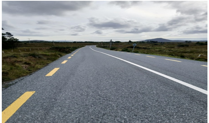
R344 INAGH VALLEY- RECENTLY SURFACE DRESSED AND LINED
