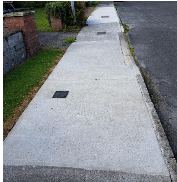
FOOTPATH REPAIRS – 16 KILGARVE COURT, BALLINASLOE TOWN
