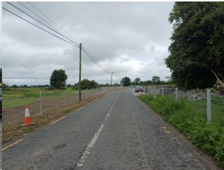
R350 BULLAUN ROAD – ERECTION OF POST AND WIRE FENCING
