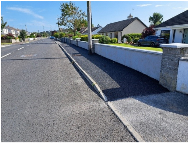
FOOTPATH REPAIRS – DERRYMULLEN, BALLINASLOE TOWN
