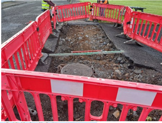
FOOTPATH REINSTATEMENT, BEECHGROVE, ORANMORE
