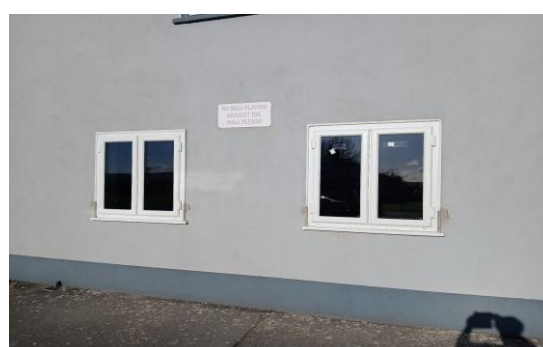
Leitrim Ballydugan Community Centre & Field – replaced windows
