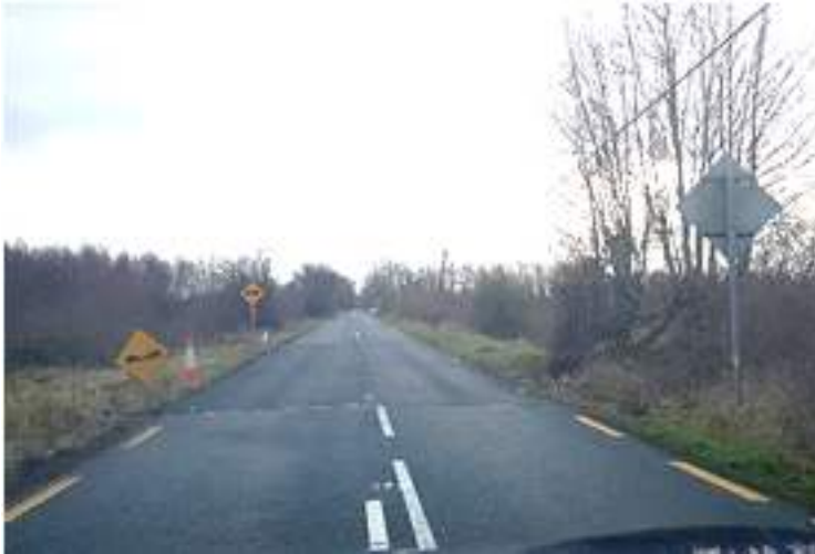
..... AFTER ROAD REPAIRS N83 DUNMORE TO CLOONFAD ROAD
