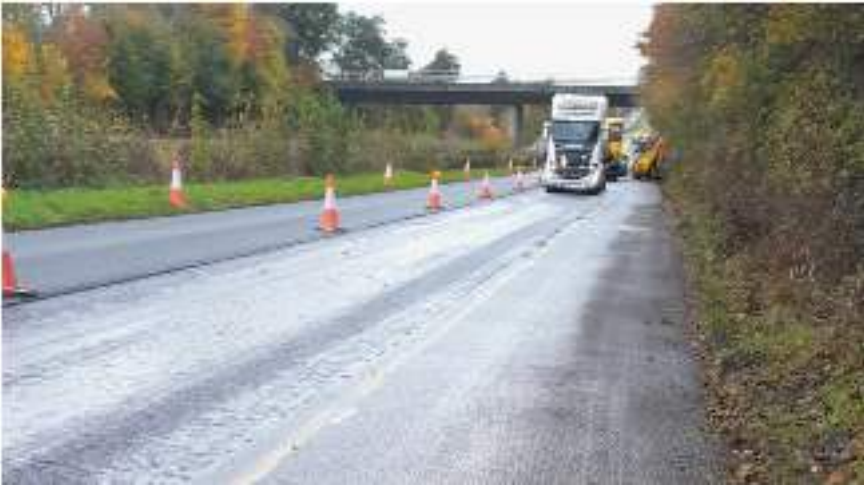
R446 DUAL CARRIAGEWAY WORKS – COMPLETE
