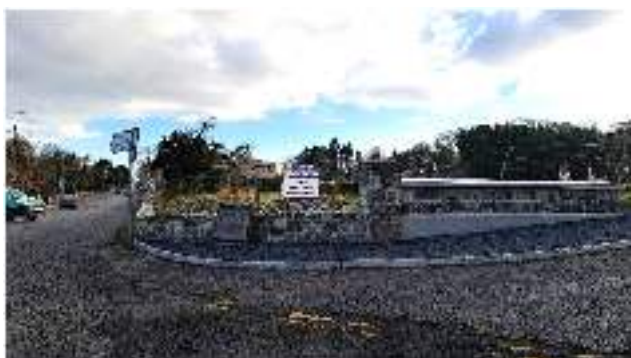
CIS SCHEME AT DÚN ÍDE ESTATE ENTRANCE, BALLINASLOE R348 - SIGHTLINE SAFETY WORKS COMPLETE DECEMBER 2023
