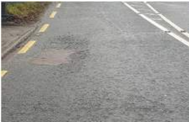
..... BEFORE ROAD REPAIRS N83 DUNMORE
