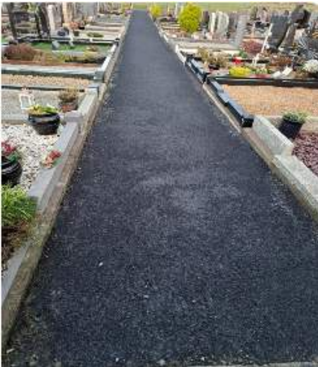
CEMETERY FOOTPATH UPGRADE WORKS – RENVILLE
