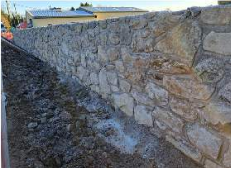
CONSTRUCTION OF A STONE WALL IN LABANE TO FACILITATE A NEW FOOTPATH.
