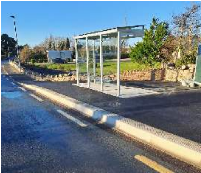
NEWLY INSTALLED BUS SHELTER CASLA
