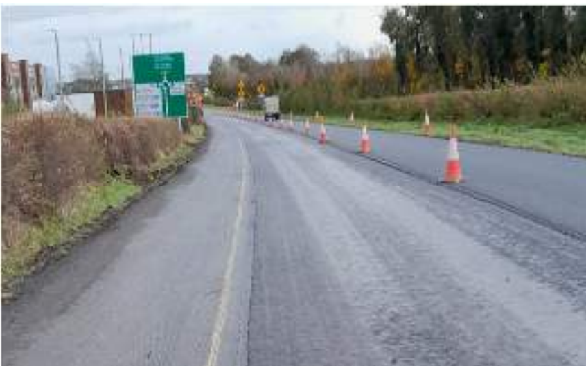
R446 DUAL CARRIAGEWAY WORKS – COMPLETE
