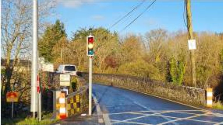
CREGMORE BRIDGE LIGHTS REPAIR
