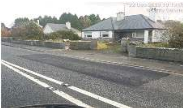
..... AFTER ROAD REPAIRS N83 DUNMORE
