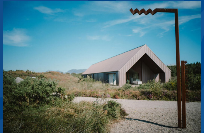
Ionad Cultúrtha an Phiarsaigh, Pearse Cottage, Visitor Centre, Connemara, Co. Galway.
