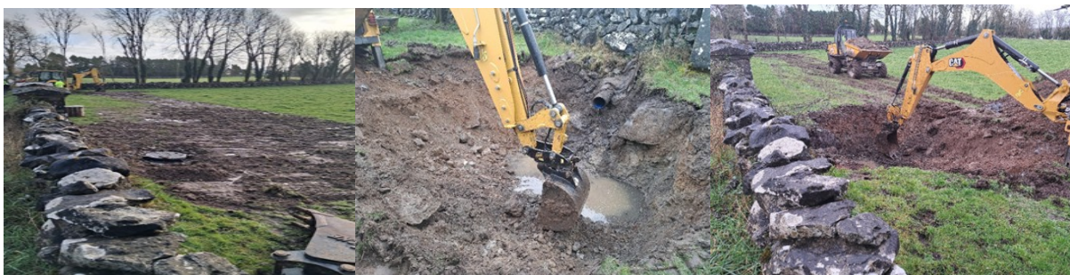
INSTALLATION OF SOAKPIT, KILLEENEEN.
