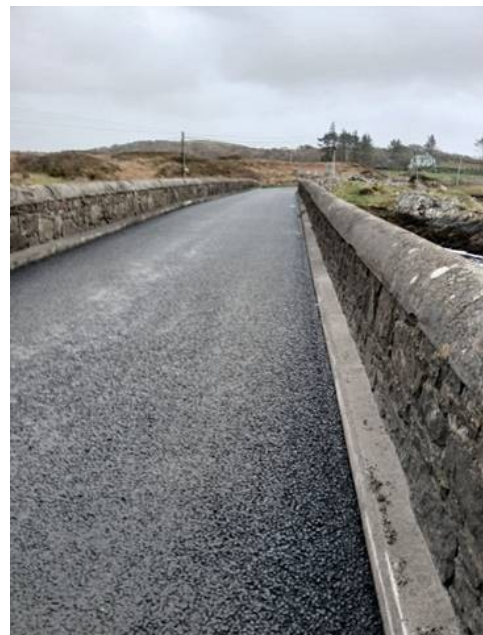
ADDITIONAL RESTORATION IMPROVEMENT PROJECT 2025 - SALT LAKE BRIDGE, R341, CLIFDEN
