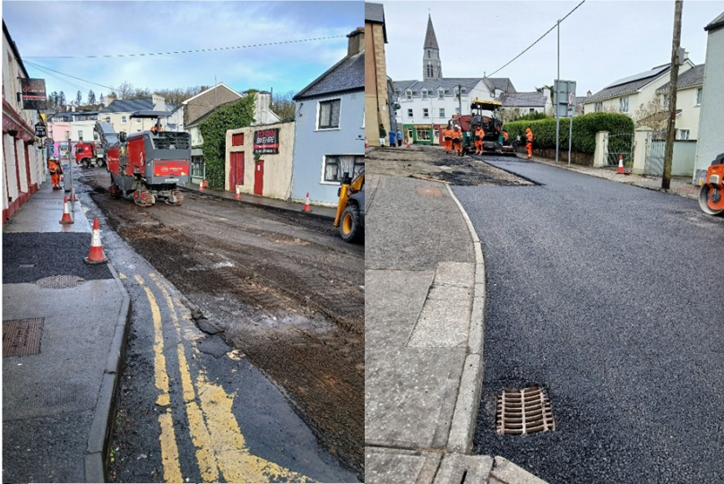
BRIDGE ST. CLIFDEN INLAY PROJECT 2025 (RESTORATION IMPROVEMENT PROGRAMME)
