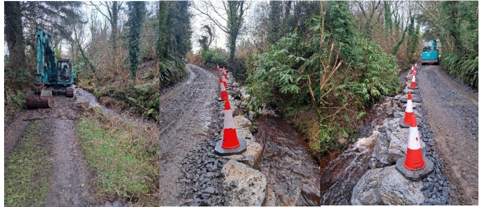
LOCALISED ROAD WIDENING AT GORTADRAGAUN.
