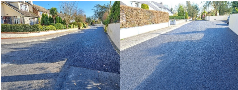
RESURFACING WORKS AT KILGARVE GARDENS, BALLINASLOE
