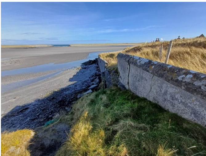
REILIG CHILL ÉINDE PERIMETER, INIS MÓR - PERIMETER WALL REPAIR PROJECT
