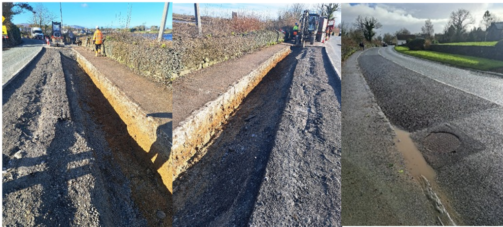
REPAIRS TO N67, KINVARA.
