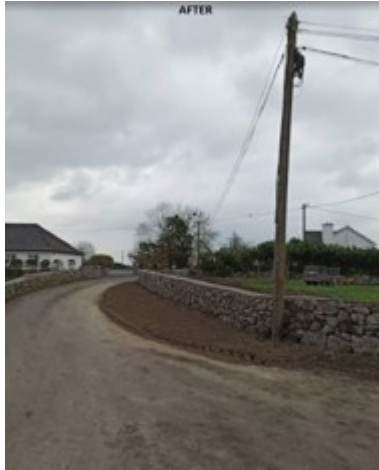
COMPLETION OF SETTING BACK WALL @ CLOCMAL.
