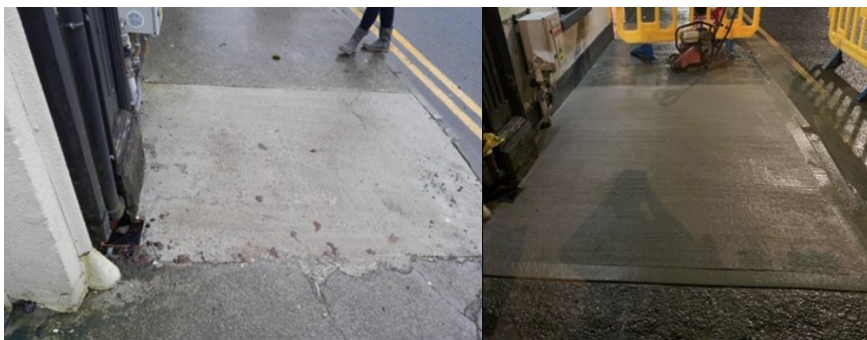
FOOTPATH REPAIRS, BRIDE STREET, LOUGHREA
