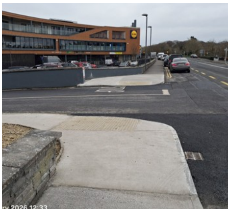
ENTRANCE IMPROVEMENT WORKS @ LIDL, ORANMORE
