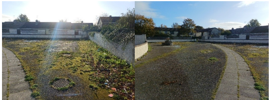
REHABILITATION OF A TARMAC PLAY AREA AT HYMANY PARK ESTATE, BALLINASLOE
