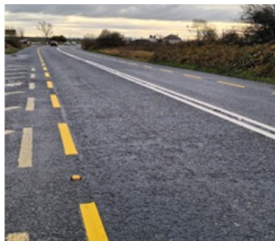
LINE REPLENISHMENT & STUD REPLACEMENT ON R354 APPROACHING CARNMORE CROSS
