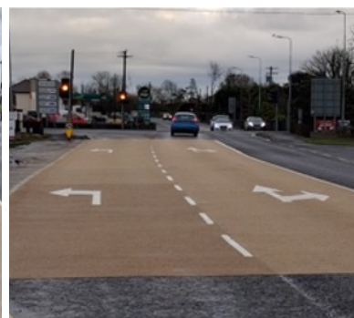
LINE REPLENISHMENT & STUD REPLACEMENT ON R354 APPROACHING CARNMORE CROSS
