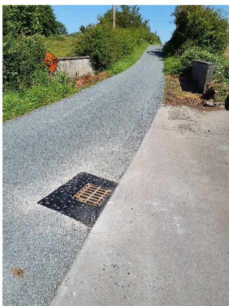
SURFACE DRESSING & DRAINAGE IRONWORKS COMPLETED AT FAHY (LEFT)
