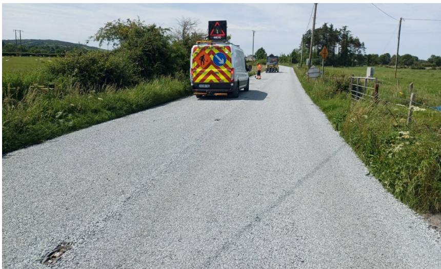
EXPOSING ROAD STUDS ("CATS EYES") POST SURFACE DRESSING ON R380
