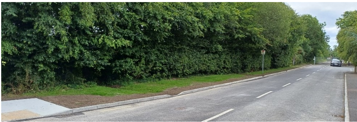
NEW ROAD EDGE KERBING COMPLETED AT HILLCREST (ABOVE)
