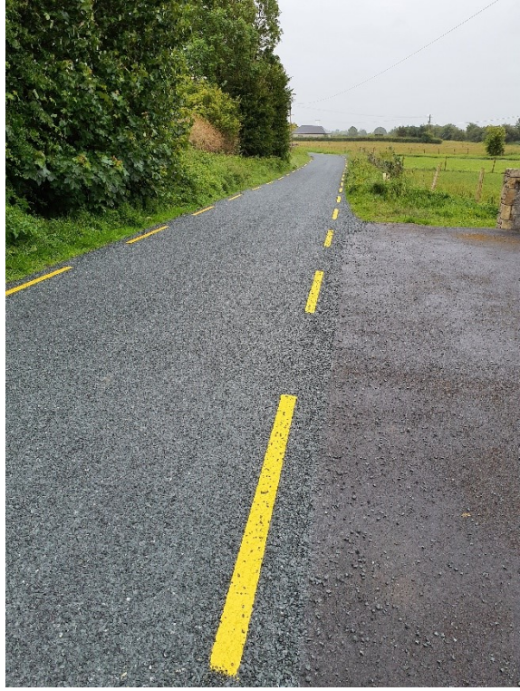
CLONBROCK – (RM) SURFACE DRESSING & LINE MARKING – WORKS COMPLETED
