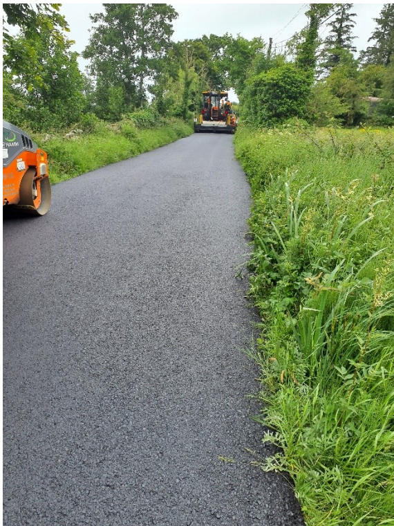
MILFORD – (RI) DBM STRENGTHENING WORKS UNDERWAY (IN ADVANCE OF FINAL SURFACE DRESSING COURSE)
