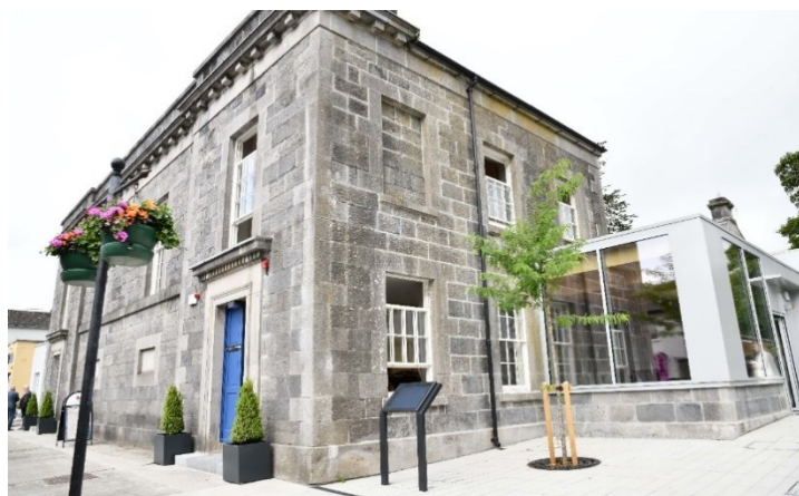
PORTUMNA COURTHOUSE THE MORNING OF THE OFFICIAL OPENING
