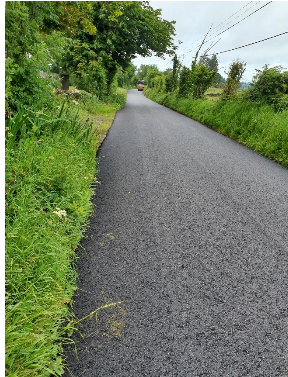
MILFORD – (RI) DBM STRENGTHENING WORKS UNDERWAY (IN ADVANCE OF FINAL SURFACE DRESSING COURSE)
