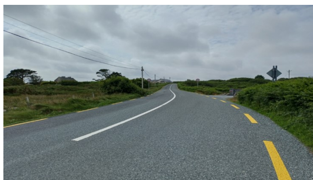
R374, AN LEIC NEAR LEITIR MÓIR - RECENTLY SURFACE DRESSED AND LINED
