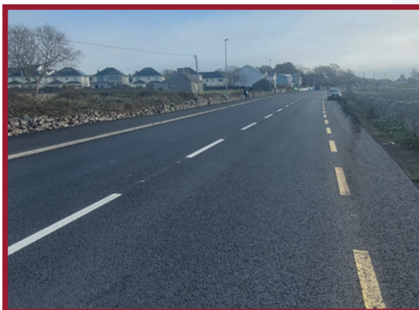
Coast Road Oranmore Footpath and Roadworks
