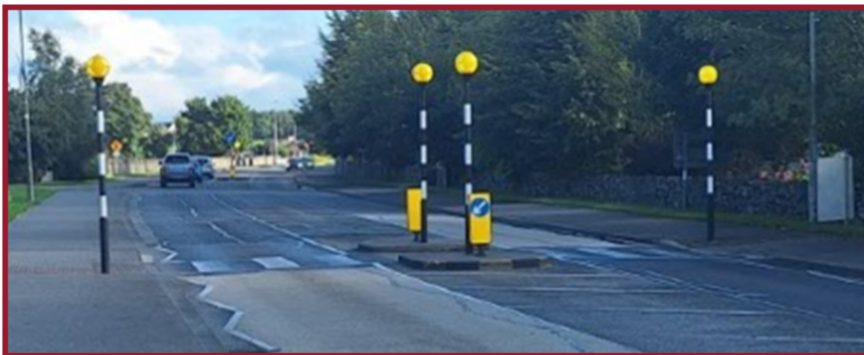
NS New Pedestrian Crossing Lights
