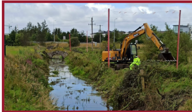
Lavally Drainage District Works – Athenry River Cleaning
