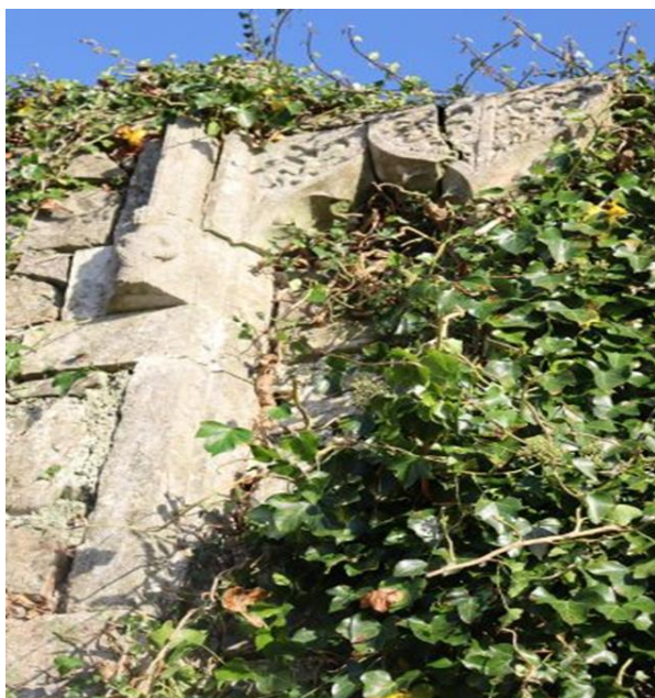
ST. KERRILL'S OGEE HEADED WINDOW, UNDER IVY AND EXTREMELY FRAGILE BEFORE CONSERVATION (2023)
