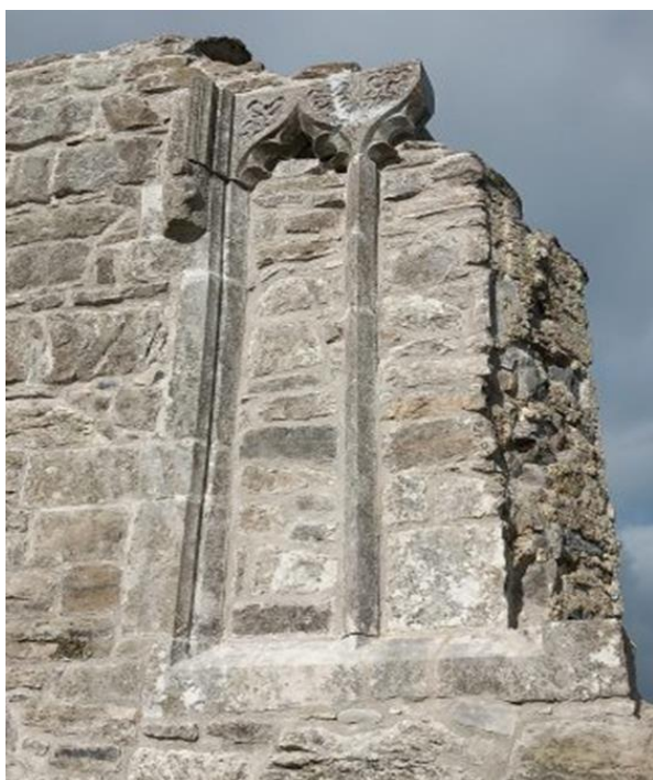
ST. KERRILL'S OGEE HEADED WINDOW, AFTER RECONSTRUCTION (2023)
