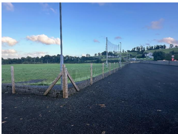
New fencing and gates at Ballinakill Sportsfield, Loughrea
