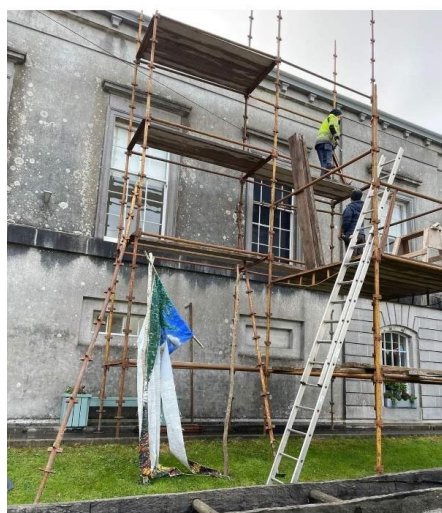
Roof repairs at Oughterard Courthouse in Oughterard
