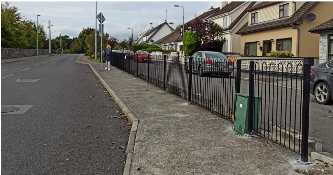
ARD AOIBHEANN RAILING
