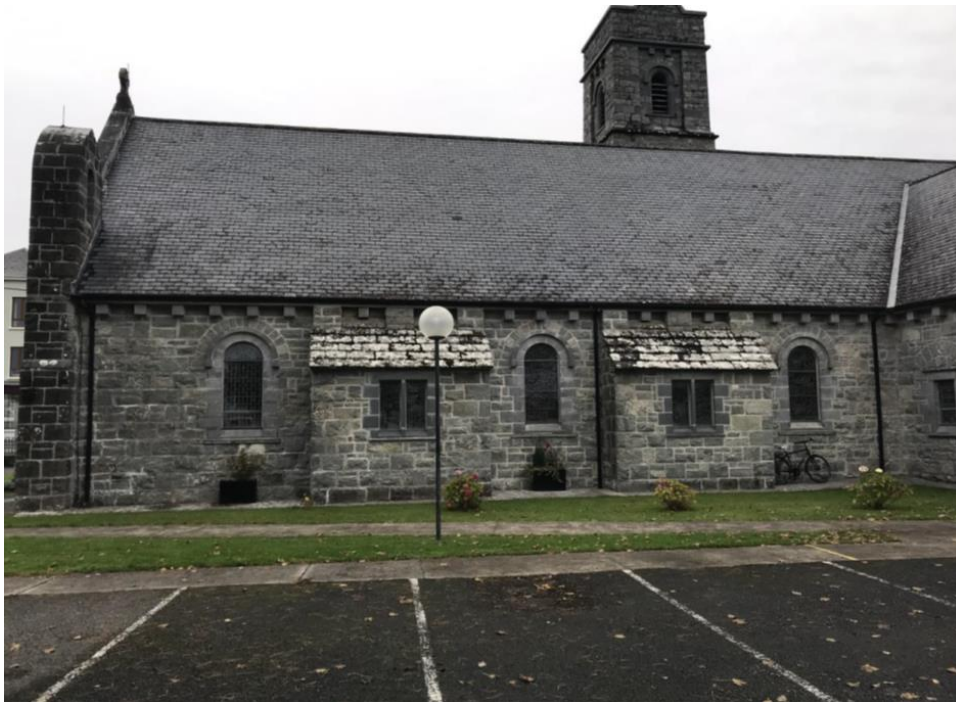
CILL EINDE, AN SPIDÉAL. REPAIRS TO SOUTH FAÇADE POINTING AND TO RAINWATER GOODS.
