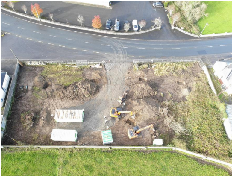
AERIAL VIEW OF SITE CLEARANCE WORKS AT BALLYMOE
