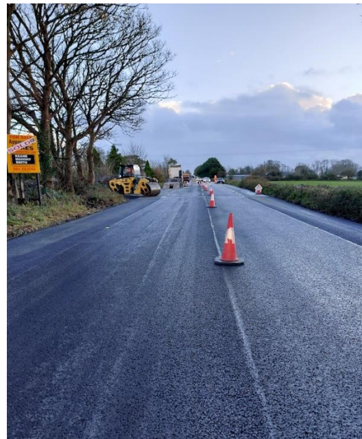
Completion of works
