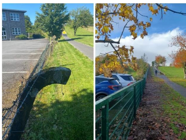
FENCING UPGRADE FOR THE PALACE GROUNDS
