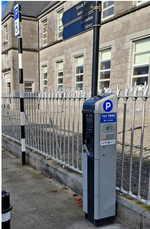
INSTALLATION COMPLETED OF REPLACEMENT SOLAR POWERED PARKING TICKET MACHINES IN BALLINASLOE TOWN.
