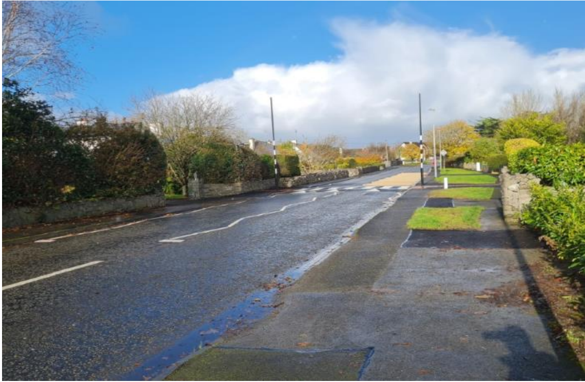
MAREE ROAD PEDESTRIAN CROSSING
