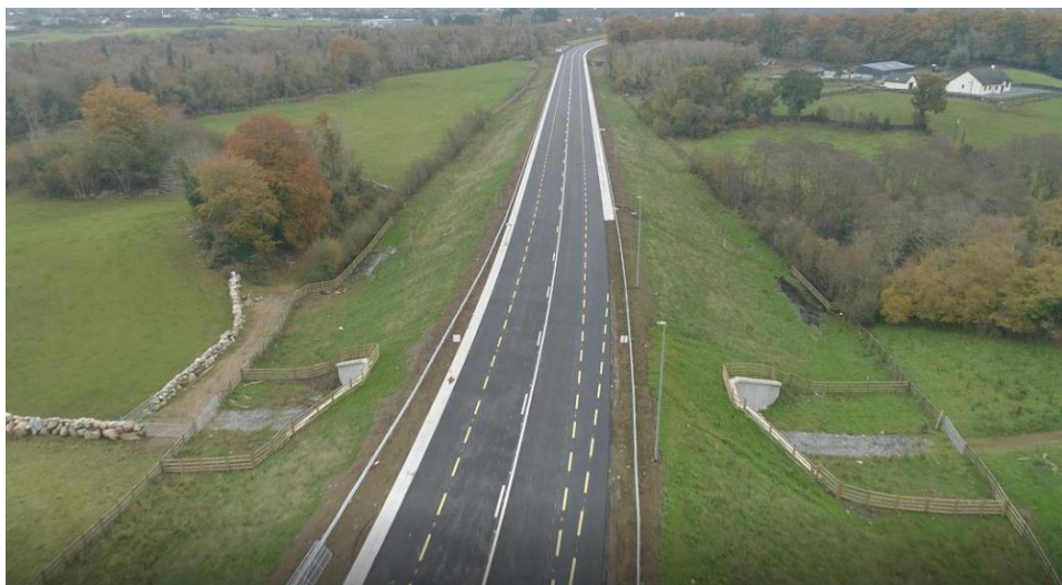
N59 MOYCULLEN BYPASS MAINLINE.
