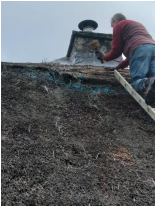
REPAIR TO COMB AND APPLICATION OF BLUESTONE TO THATCH NEWTOWNSMITH, DURUS, KINVARA BHIS 2023
