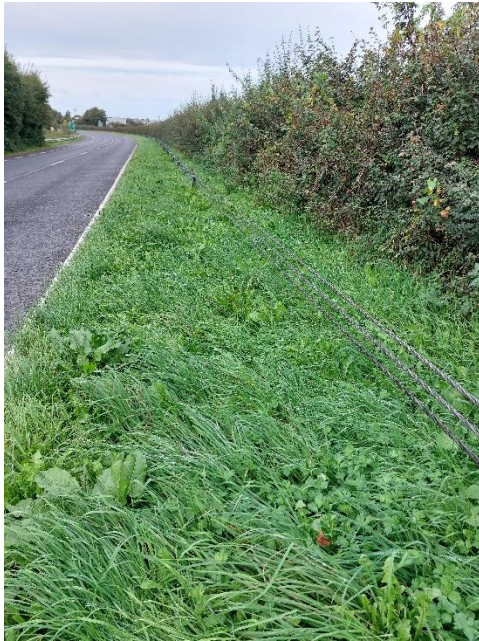
Damaged barrier
