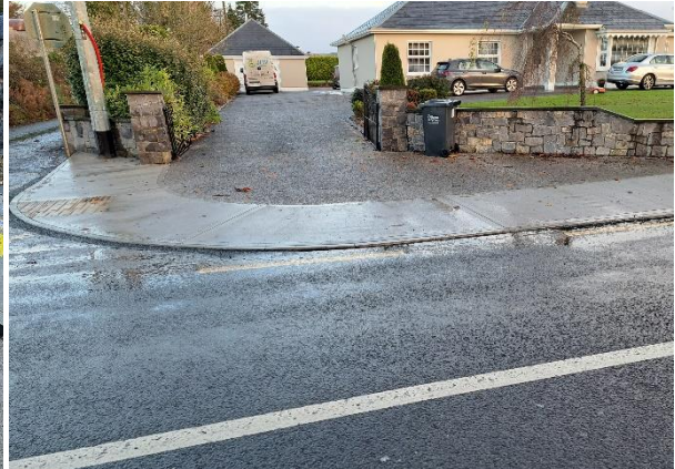
COMPLETED FOOTPATH & PUBLIC LIGHTING CONSTRUCTION WORKS AT AHASCRAUGH ON THE CALTRA ROAD R358, FUNDED UNDER THE COMMUNITY INVOLVEMENT SCHEME, PROVIDING SAFE PEDESTRIAN ACCESS.
