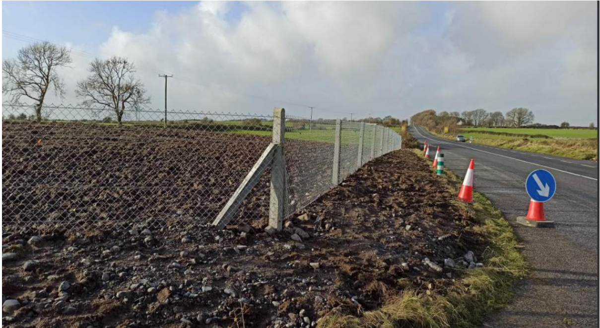
MOYVEELA JUNCTION UPGRADE
