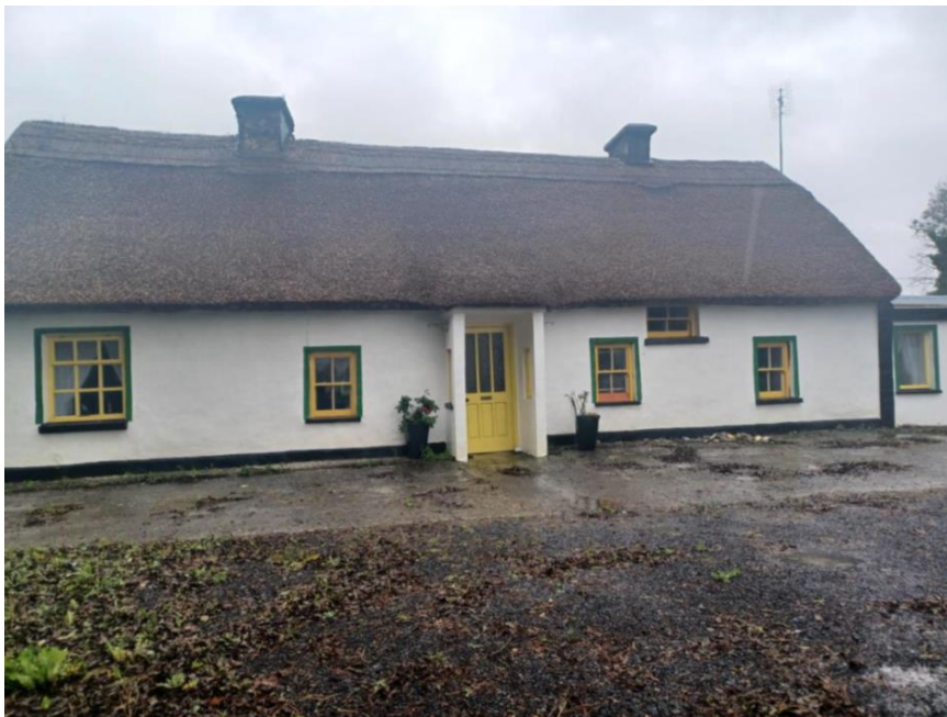
KEANE'S HOUSE; REPAIR TO WINDOWS 2023
