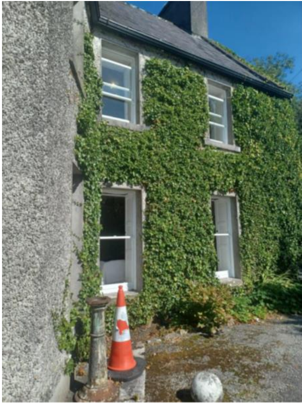
REPAIR TO TIMBER SASH WINDOWS, PROSPECT HOUSE, ATHENRY BHIS 2023
