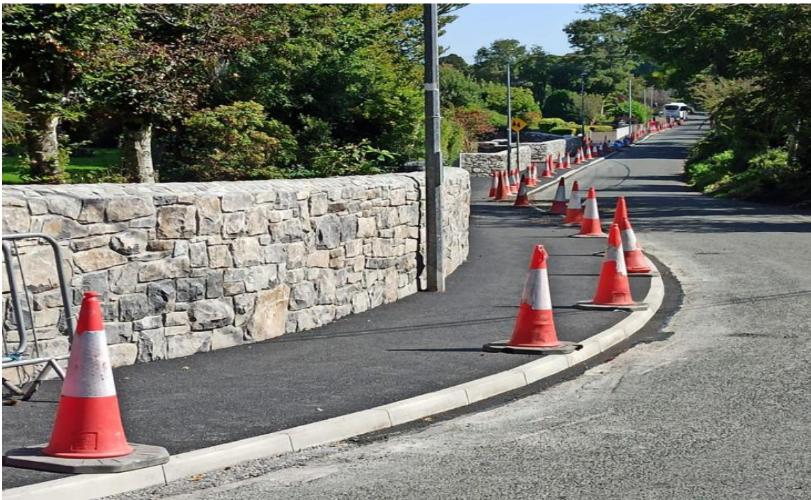
ANNAGHDOWN FOOTPATH WORKS - COMPLETE
