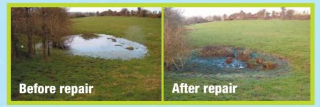
Check the ground above your pipes to look for visible signs of a leak, such as unusually damp ground.
